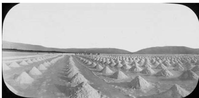
Before the salt could be transported on the tramway, it had to be harvested from the Saline Valley lake bed. Fresh water was pumped from a large spring into shallow ponds that were built on the lake bed. As the water evaporated, the salt crystals that remained were raked into piles. The salt was then shoveled into wooden railway cars that were pulled into a large storage hopper, where tramway gondolas automatically were loaded with salt. The unique system was capable of
