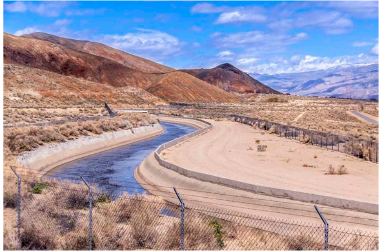
Los Angeles aqueduct. (photo courtesy of Ray DeLea)
