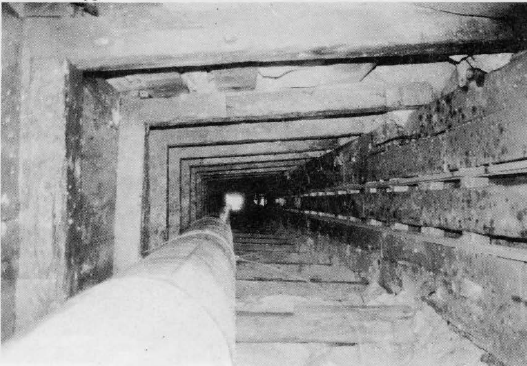
Inside the May-Lundy mine looking out. Note metal ventilator air shaft running length of tunnel. "Beware of gas."
