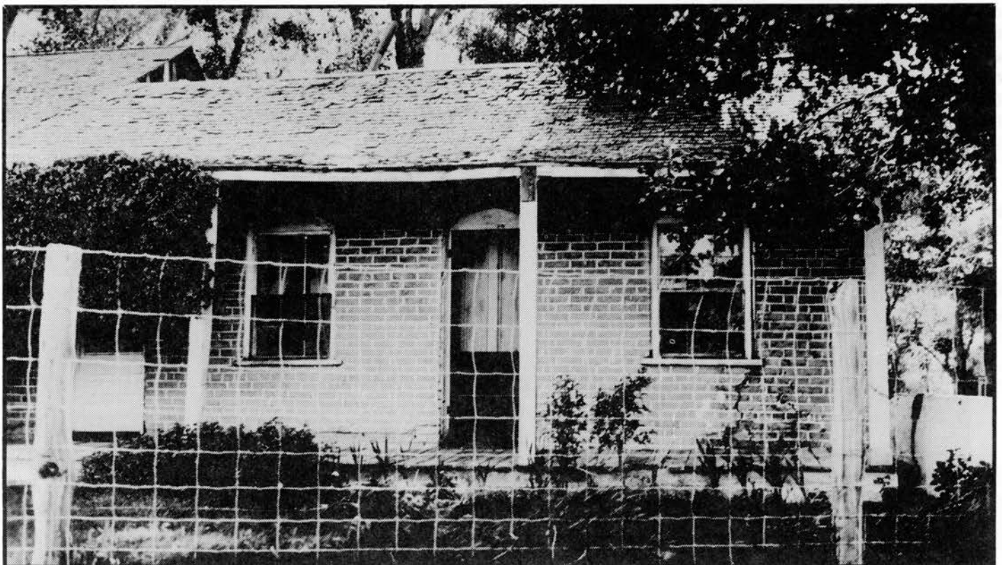
Walker House, Old Stage Station, Olancho, an adobe brick building that survived the 1872 earthquake. Note cracks under the right window. George Brown residence in the 1920s and '30s. Eastern California Museum photo
