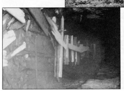
Left: View into the Sheepherder tunnel. Ore cart tracks still are spiked to their ties, but lay under six inches of running water from tapped springs in the bowels of the Sierra granite.
