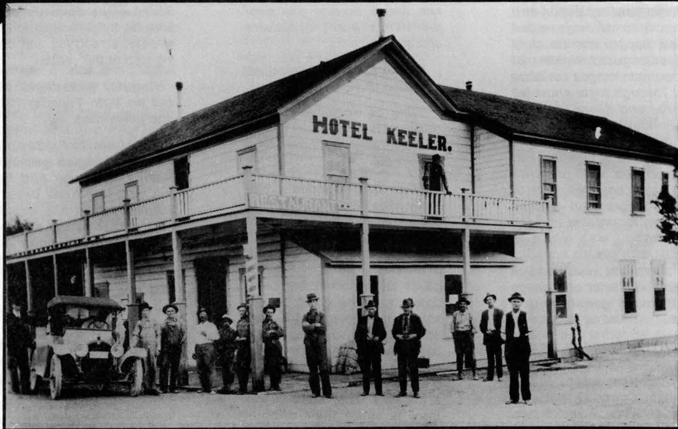
Until it burned to the ground, Hotel Keeler, operated by Mr. and Mrs. George Mates, provided for travelers at the southern terminus of the former Carson and Colorado Railroad, as well as those in the stage coaches bound for Mojave or nearby mining towns. Photo: Eastern California Museum collection.
