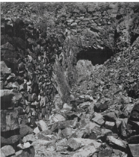
The adit of the Green Monster Mine has almost been sealed by a collapsing retaining wall. An early day [1860's] gold claim, it later produced copper.
