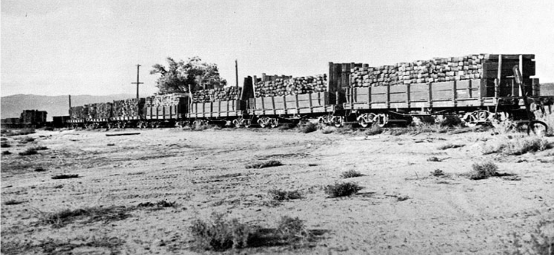
Shown is a portion of the ties removed as a result of the abandonment of the Tonopah function to Benton section during 1943.
