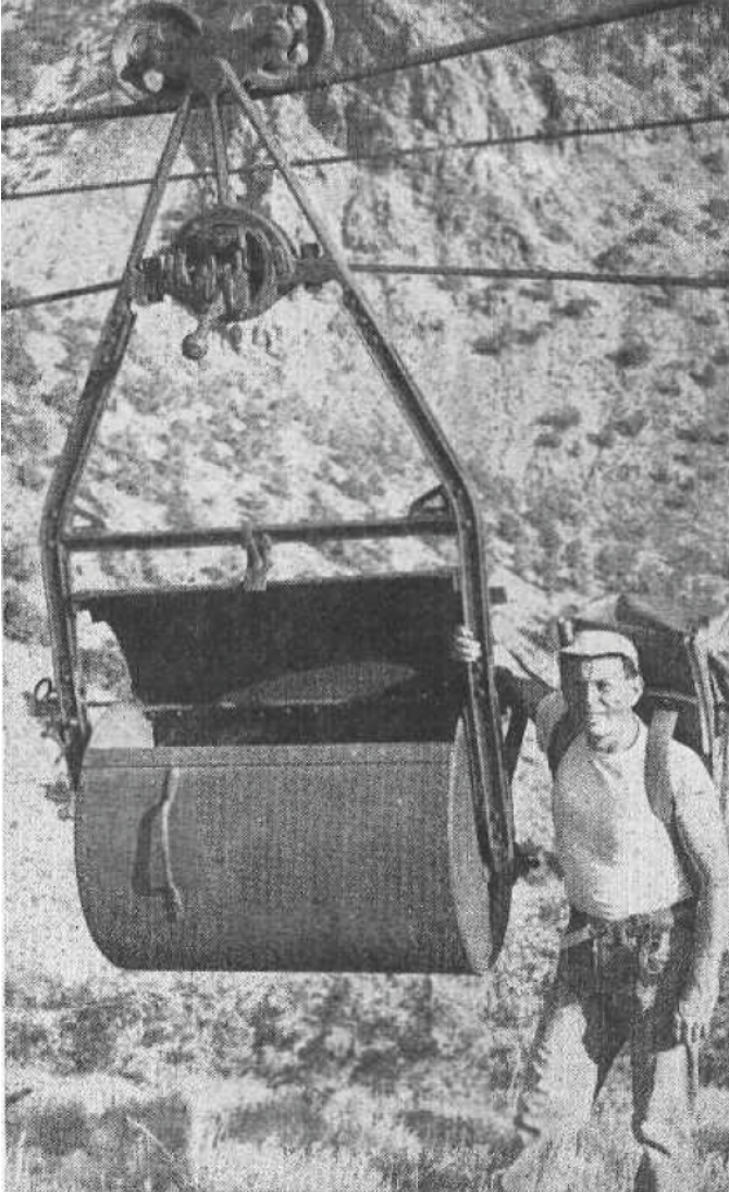
THE AUTHOR AND ONE OF THE SALINE VALLEY TRAM BUCKETS. STEEL CONTAINER HELD ABOUT 800 POUNDS OF SALT. ITS TWO-WHEEL CARRIAGE RODE THE STATIONARY SMOOTH TRACK CABLE WHILE THE AUTOMATIC GRIP BELOW ATTACHED ITSELF TO THE MOVING TRACTION ROPE.
