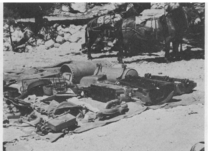
The disassembled air compressor ready to be packed on mules.
