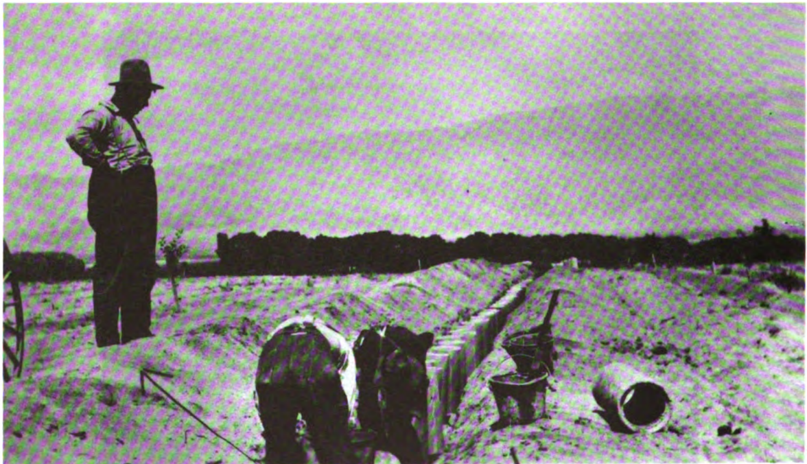
Photo 4: Van Lutzow (at left), laying cement pipe at Manzanar.
