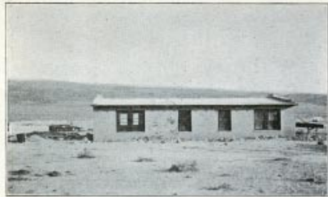
One of Our Adobe Houses Constructed of Pink Lava Clay
